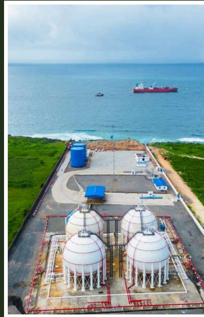
Lake Gas LPG Facility at the Industrial Park
