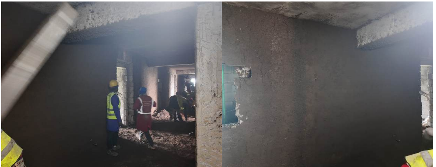
Block C Internal Plaster at level 8
