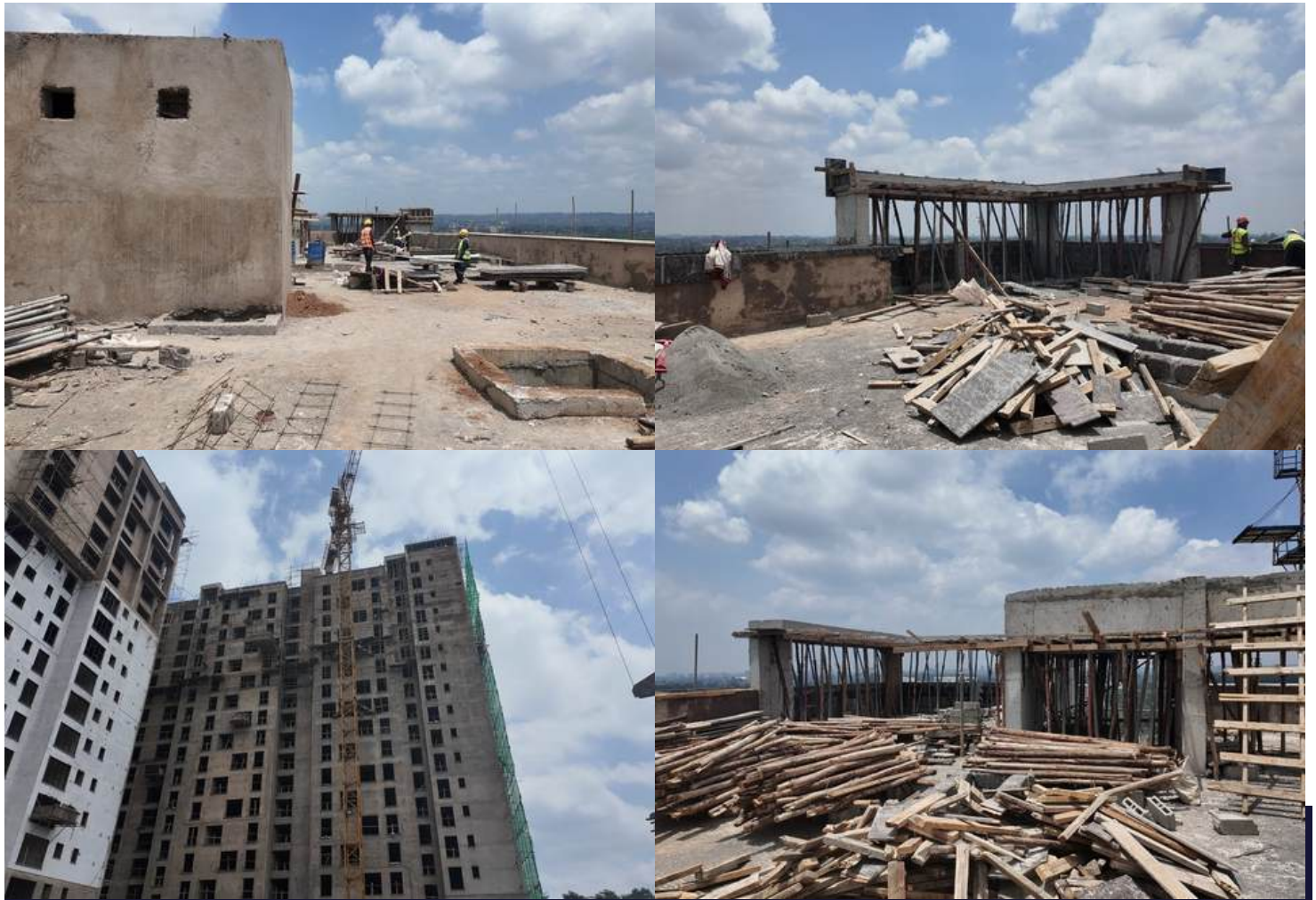
Block B Lift center beam & parapet wall coping works
