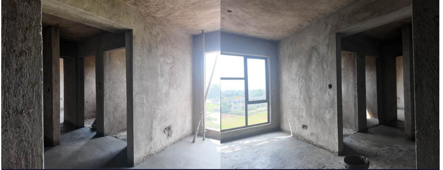
Block B Internal Plaster
