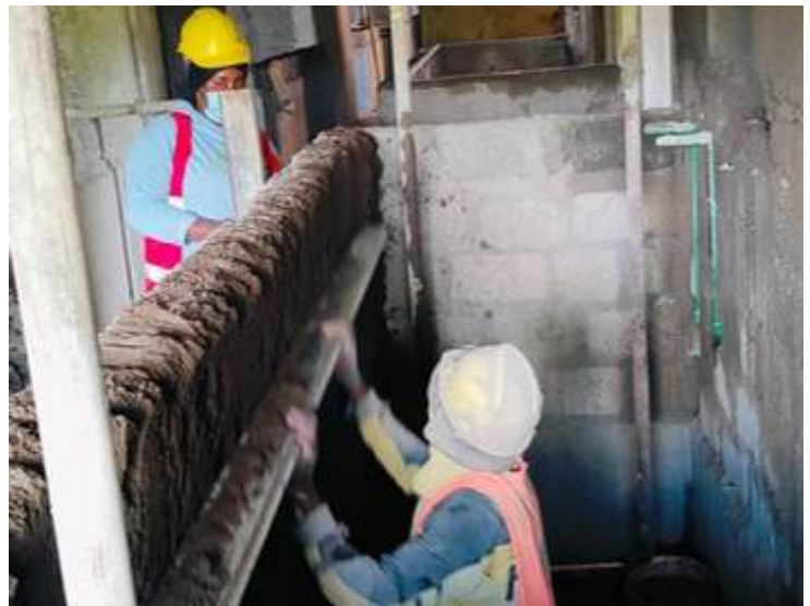
Internal Plastering
