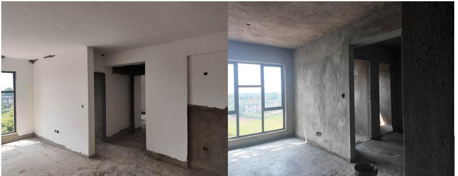
Block B Skimming and installation of door frames at level 8
