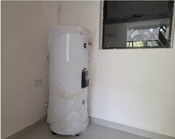
Boiler Installation
