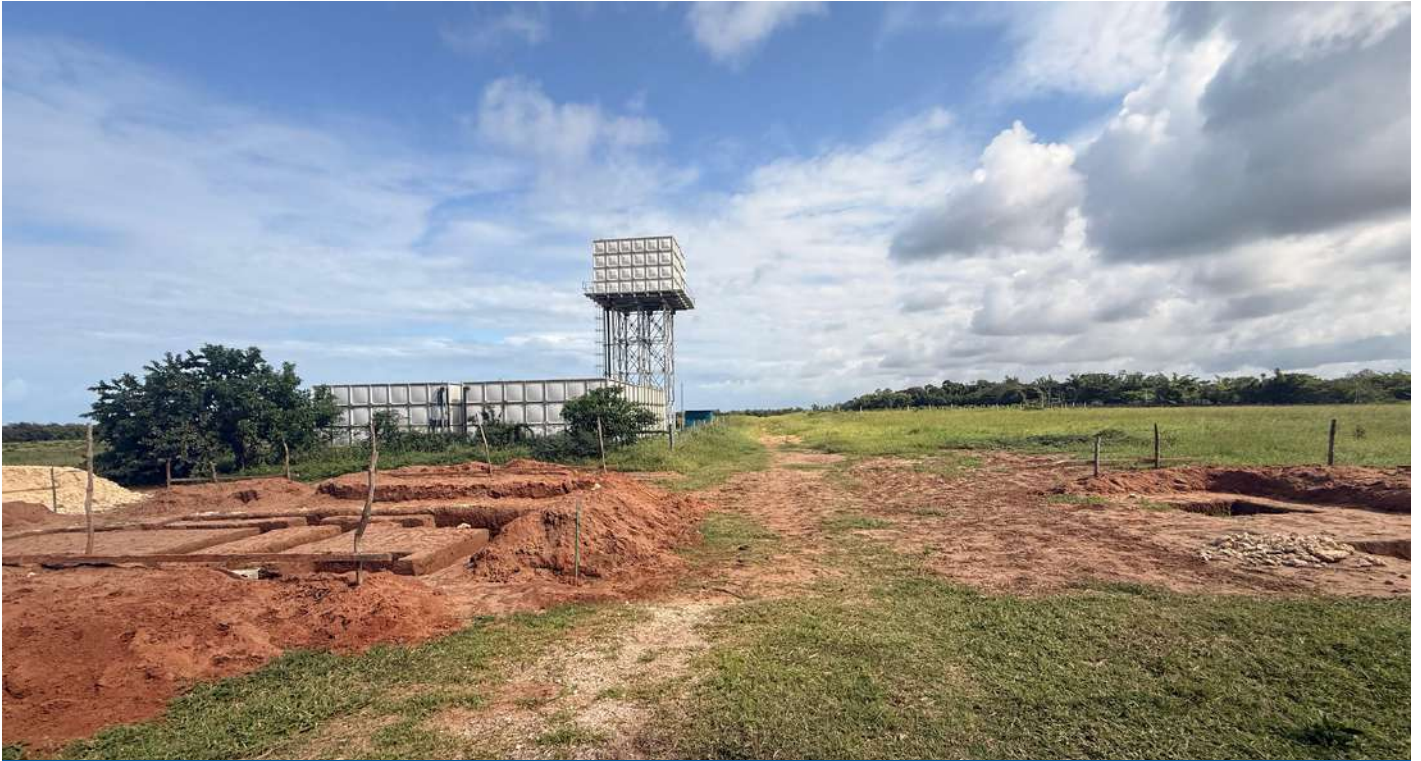
Gatehouse Foundation Excavation
