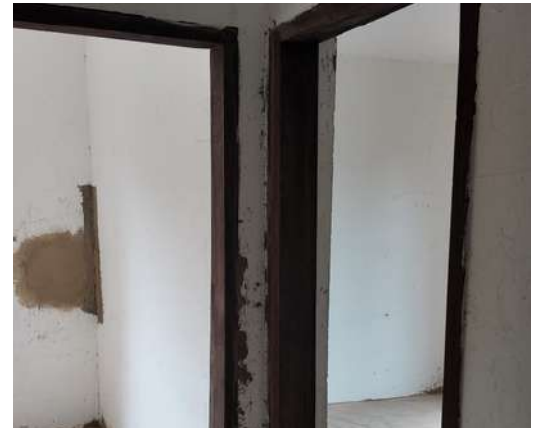
Plastering & Door Frame Installation
