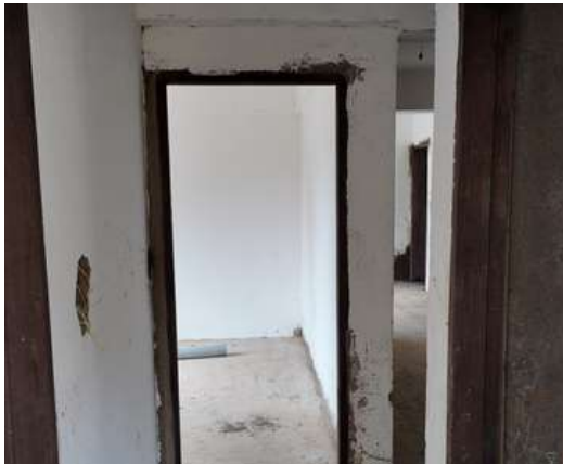
Plastering & Door Frame Installation
