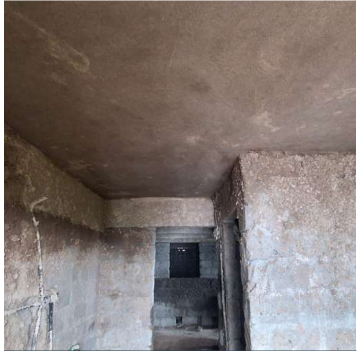
BLOCK A Level 6 & 7 Plastering
