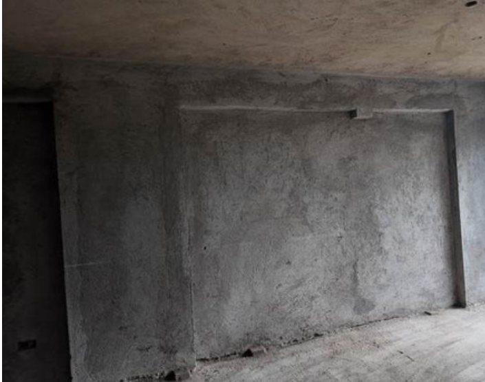
Block C Level 6 Plaster
