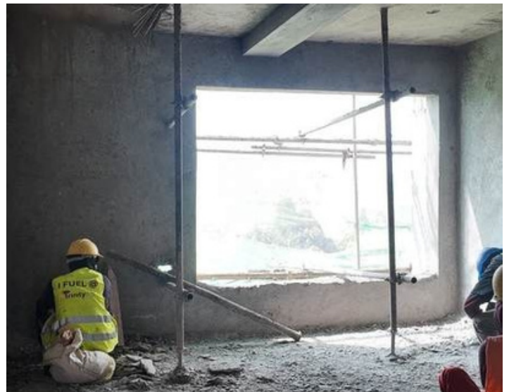
Block B Screeding
