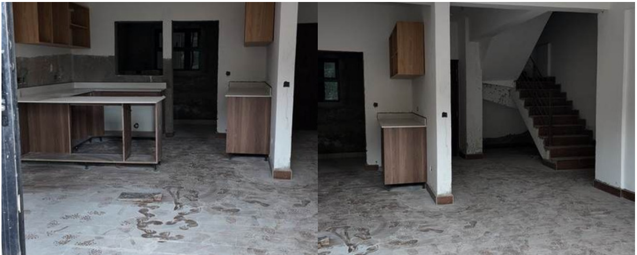
Block D & E Duplexes Floor Interior
