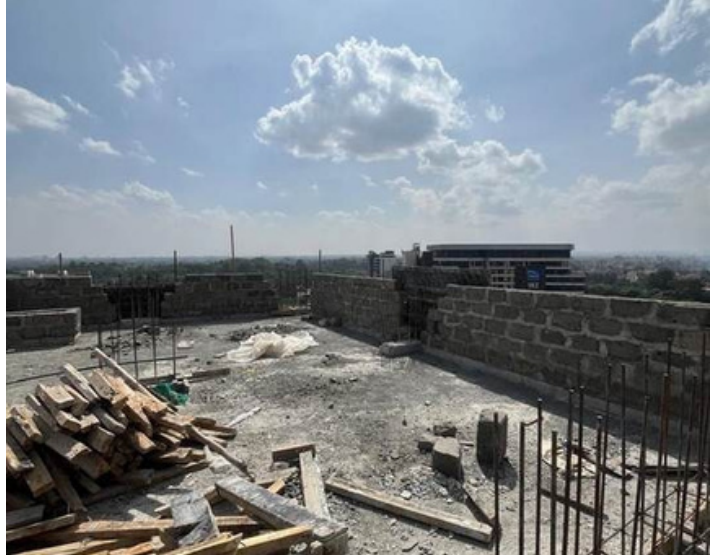
Block B rooftop walling
