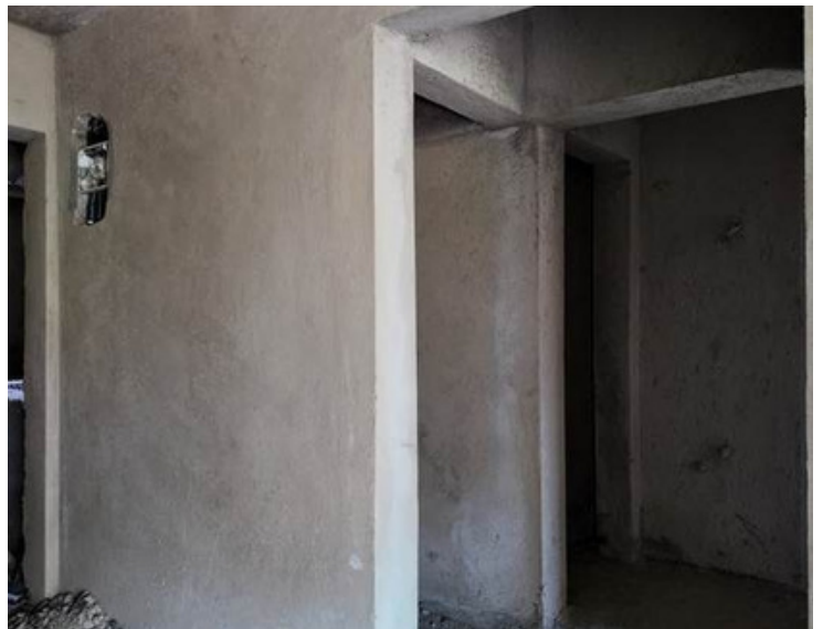
Interior Plaster Block C
