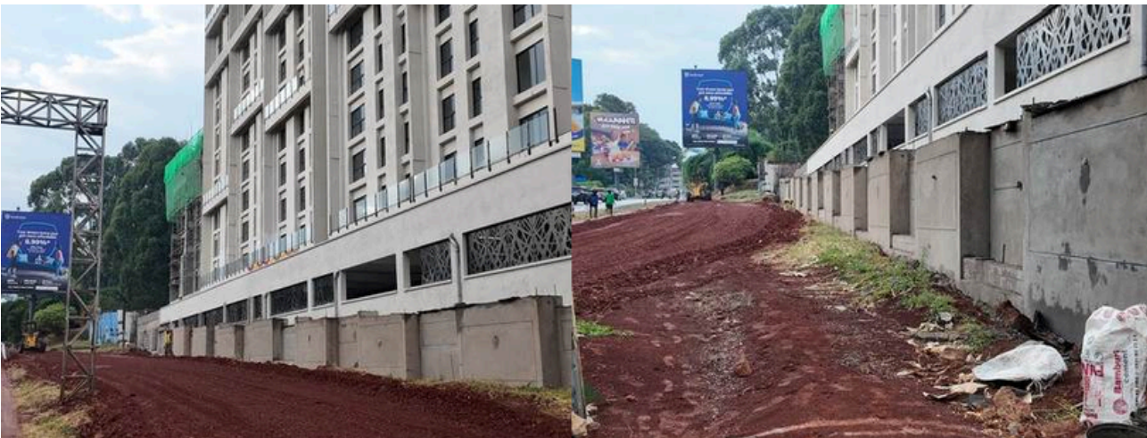
Boundary wall along Limuru road
