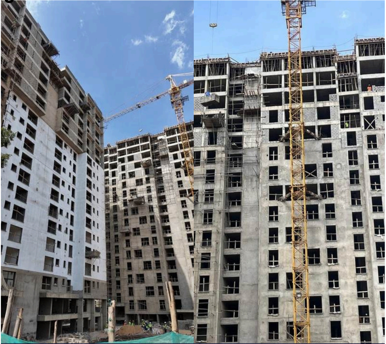
Block B & C External Plaster Ongoing
