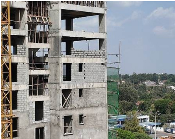
Block C Level 14 Walling Ext
