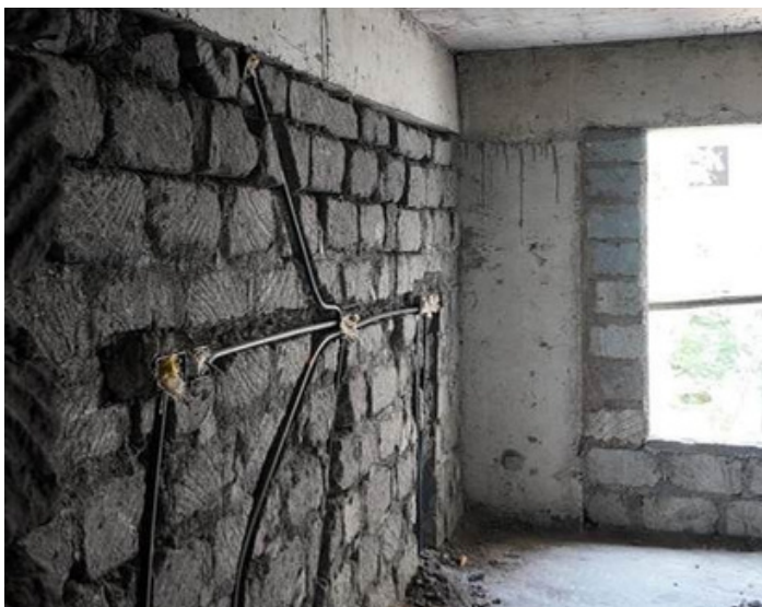
Electrical Works Block A
