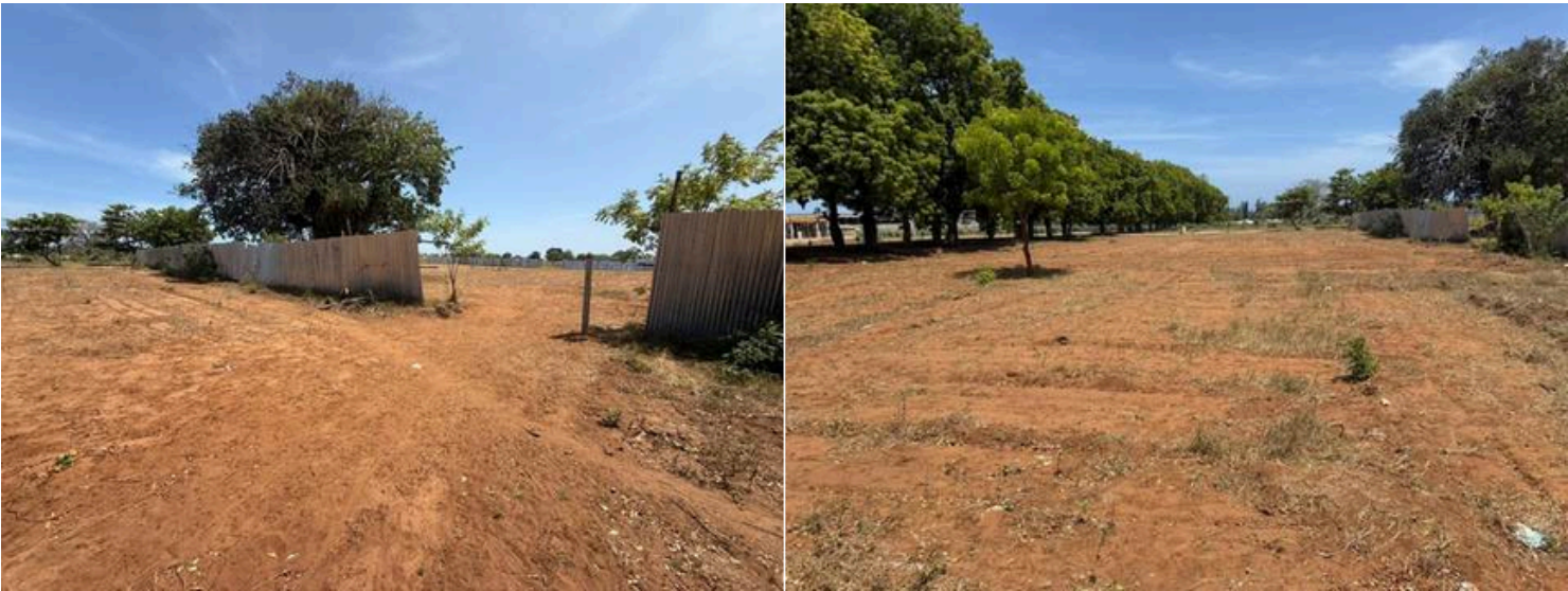
Ongoing site clearance
