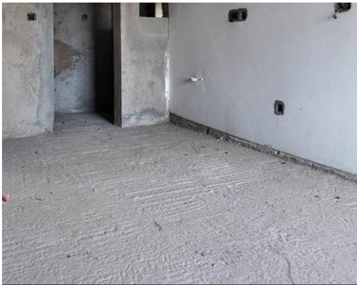
Block C Floor Hacking
