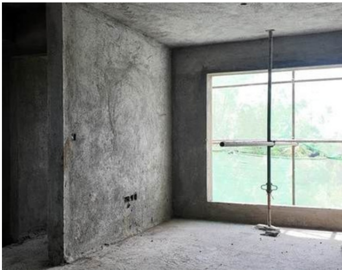
Block B 13 th Floor Internal Plaster
