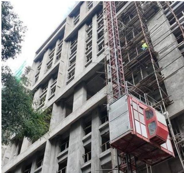
Block B Exterior Plaster
