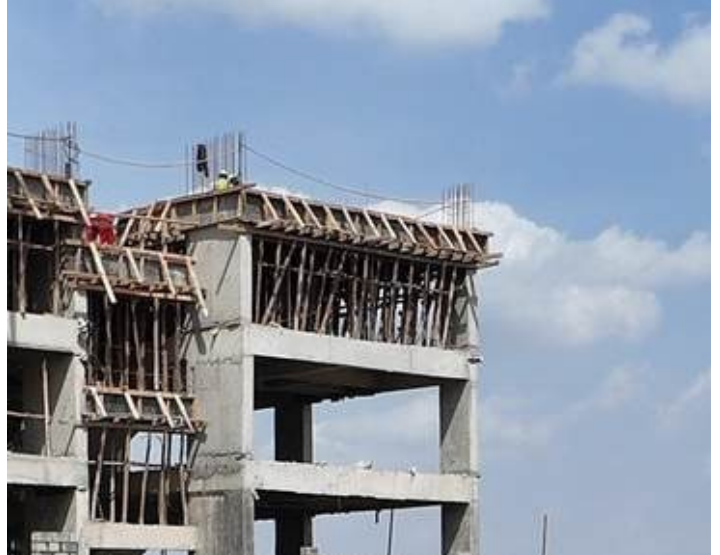
Block C Level 17 & 18 Columns
