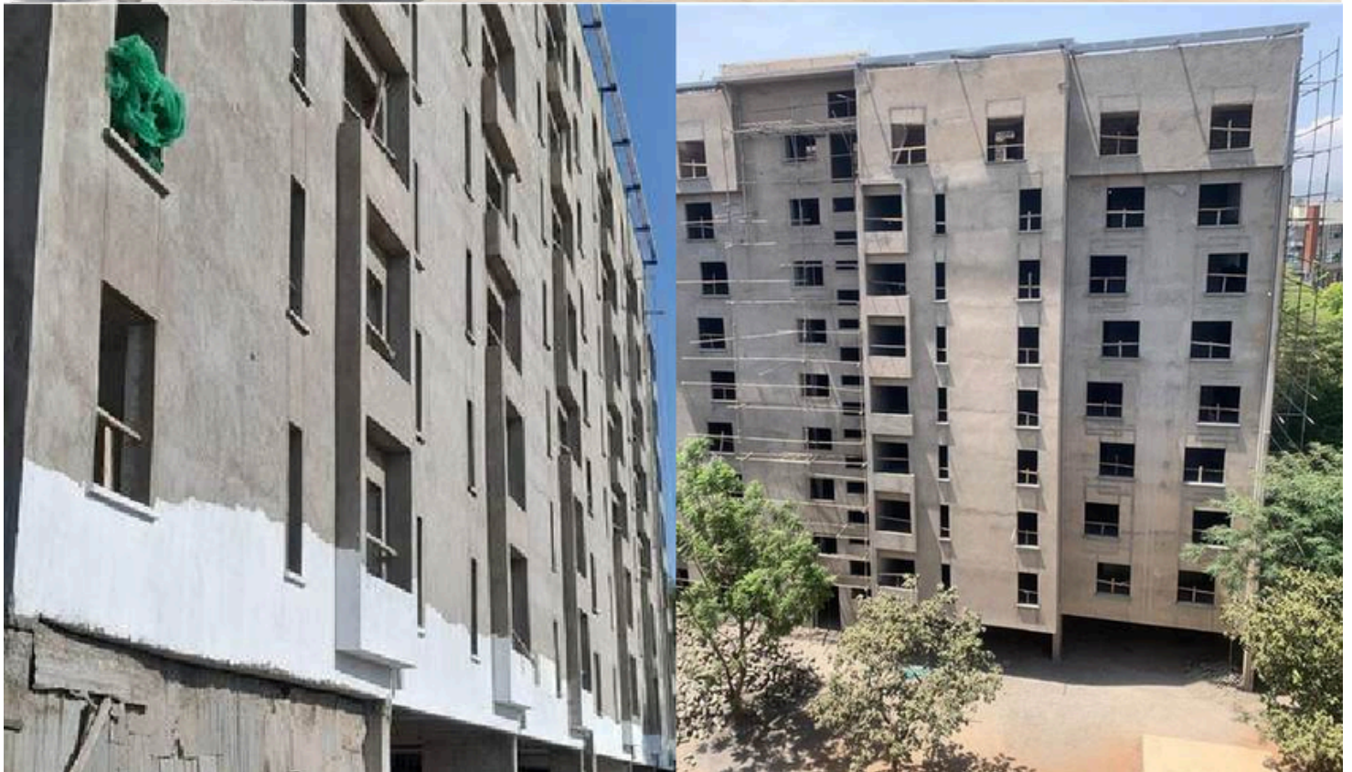
External Plaster Works
