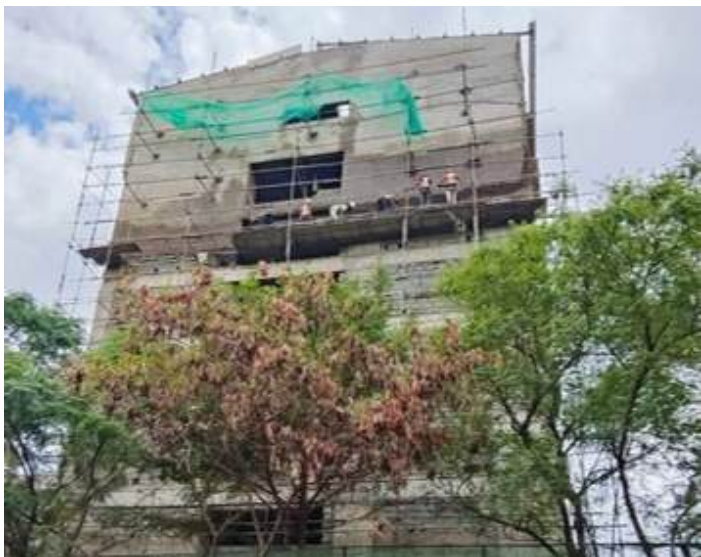
External Plaster Block A
