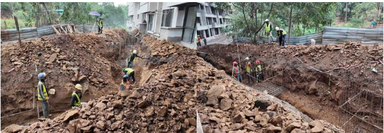
Sewer Line Works
