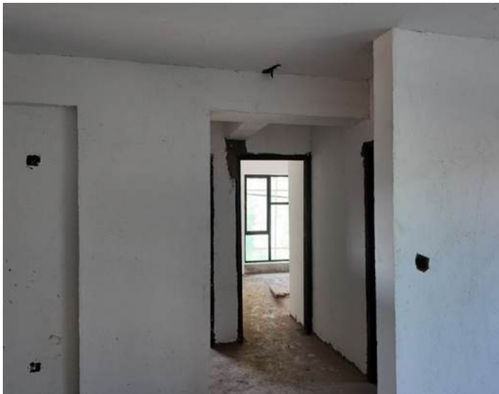
Level 5 Internal Skimming
