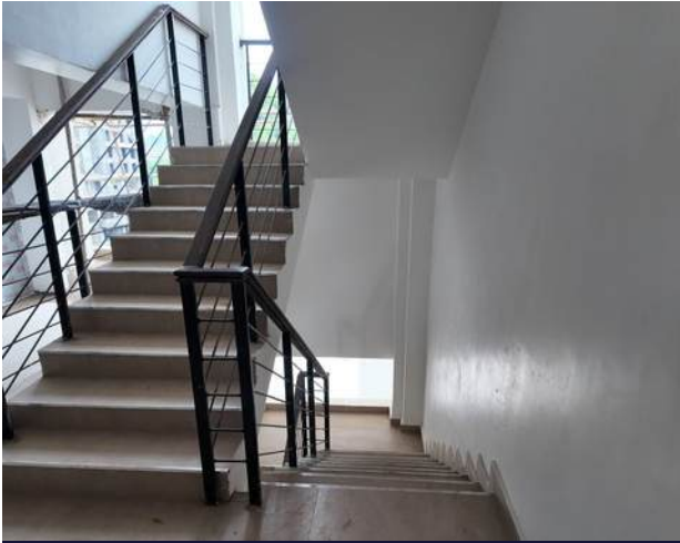
Block E Staircase
