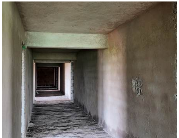
Internal Plaster Level 7
