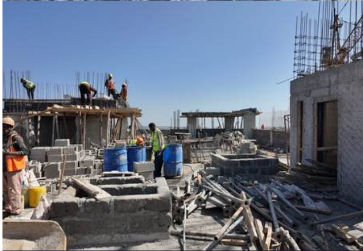
Block B Walling Ongoing at rooftop level
