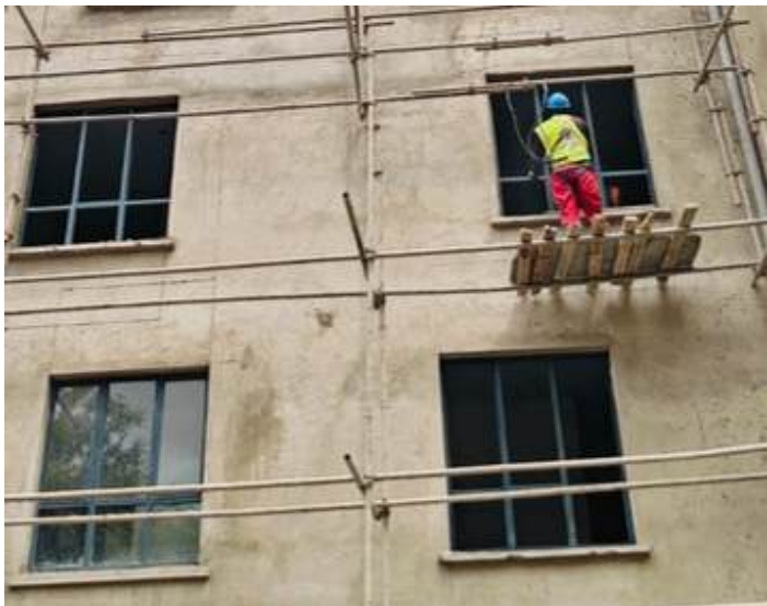
Block C Aluminium Windows Installation
