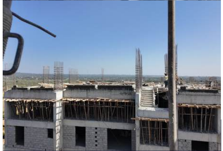
Block C Topped Out
