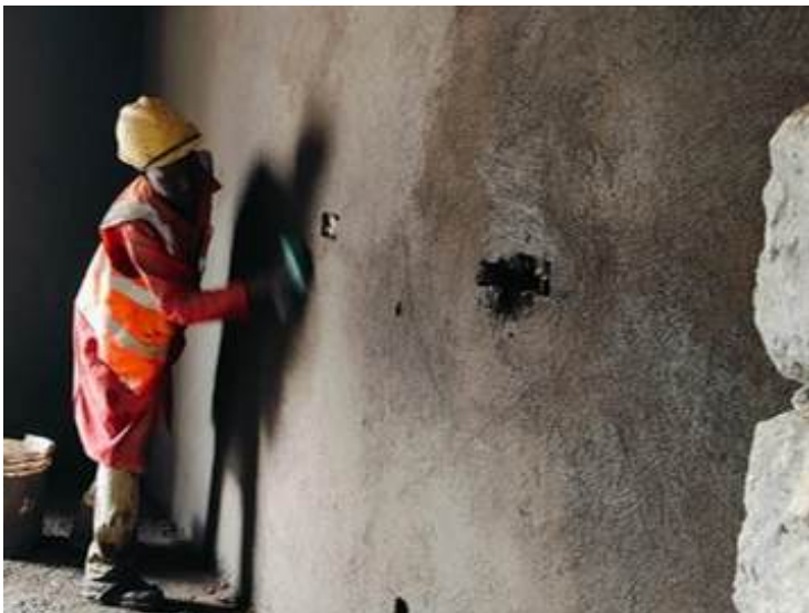
Interior Plaster Block B
