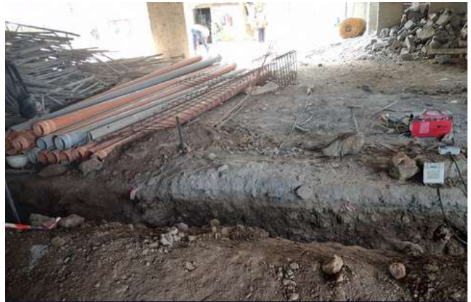
Sewerline and Boundary wall Installation
