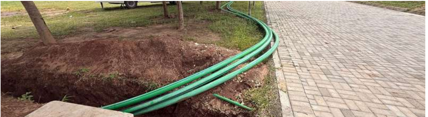
Ongoing sewer connection works at Kingswood park phase 2 & 3
