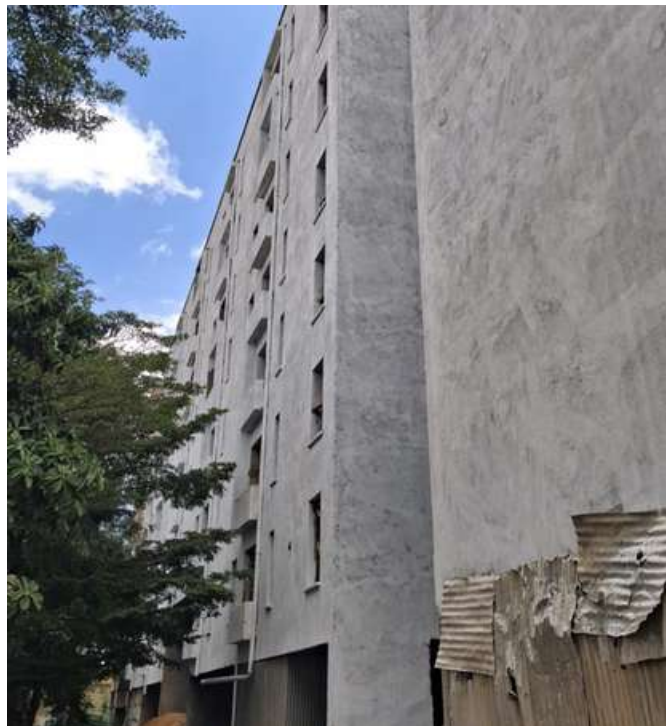
Undercoat Block B & C
