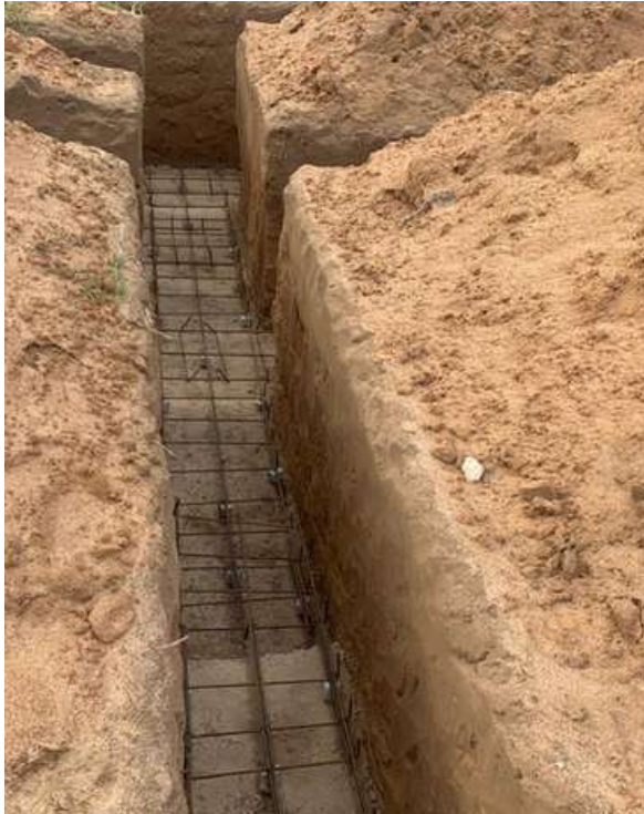
Fixing of Reinforcements in foundations
