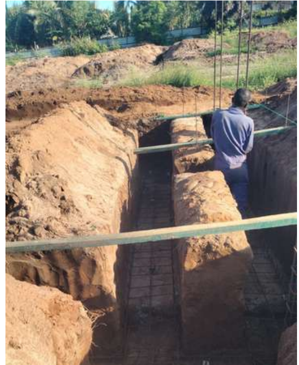
Fixing of Reinforcements in foundations
