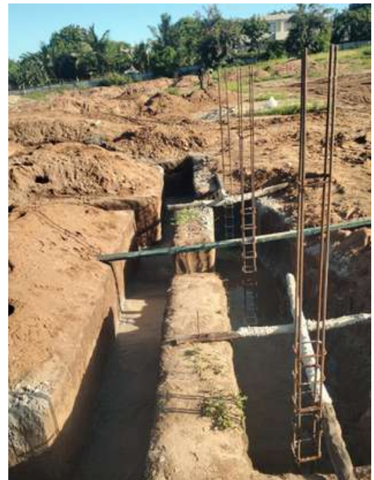
Concreting in foundations
