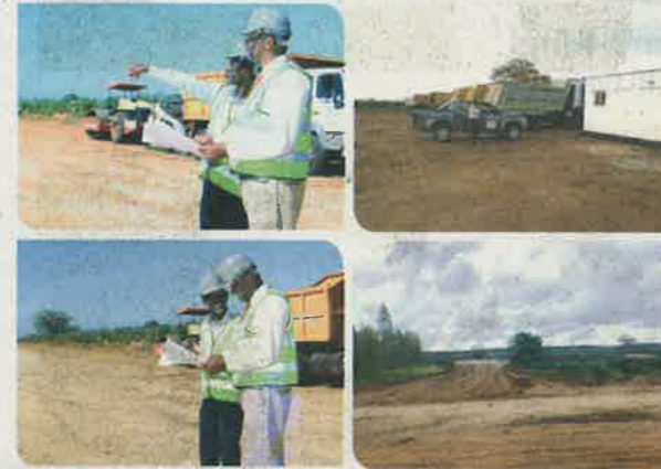
Investment Park Construction Works Ongoing
