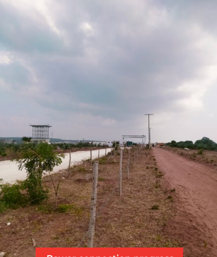
Power connection progress
